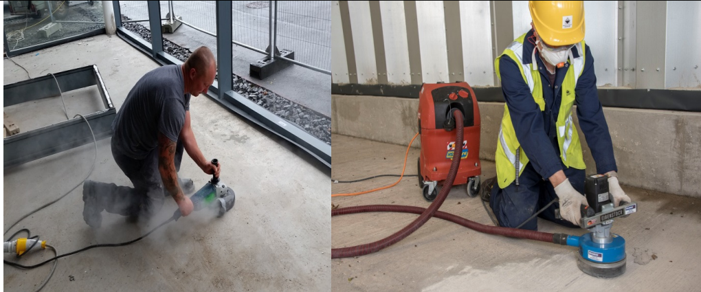
Poor Practice – Using a hand-held scabbler without on tool extraction (David Flynn Ltd, IE)
